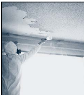
Scraping the Ceiling
