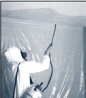
Spraying the Ceiling
